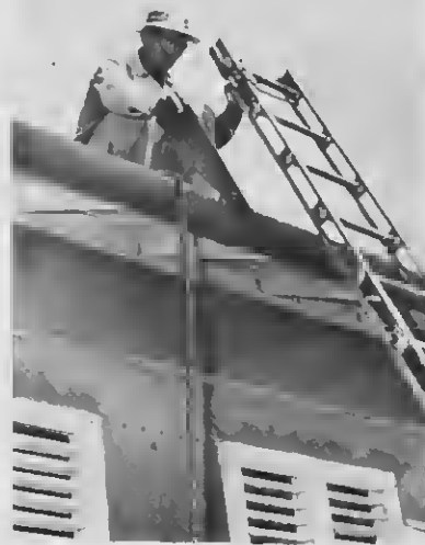
JACOBO FIGARAO , carpenter first class with over 20 years' service, starts the cut through the roof of a classroom to be moved to Santa Cruz.
